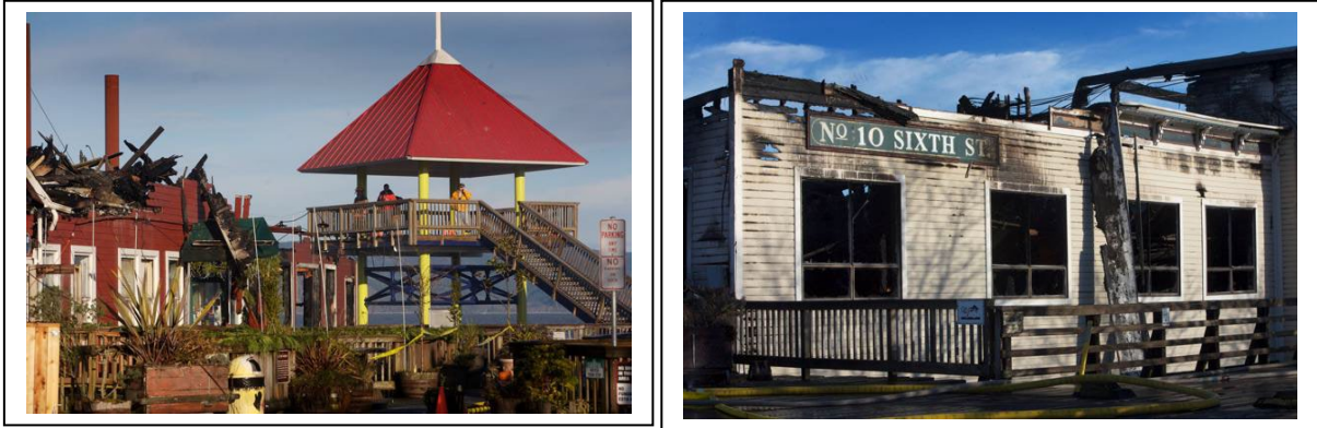
No. 10 Sixth Street fire damage
