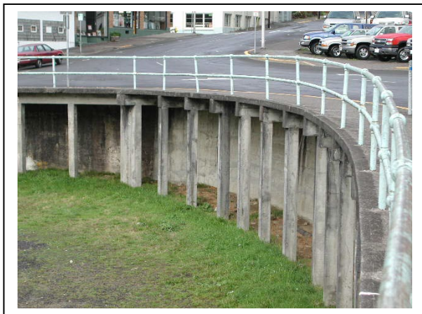
1200 Block Exchange, preserved 1923 exposed Chairwall
