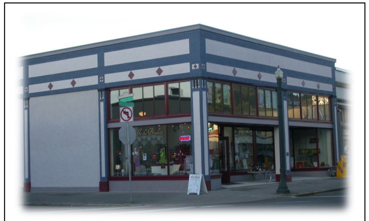
1008 Commercial, Diamond in the Rough Project
