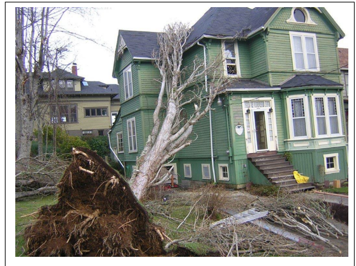
934 Irving Avenue, 2007 windstorm damage
