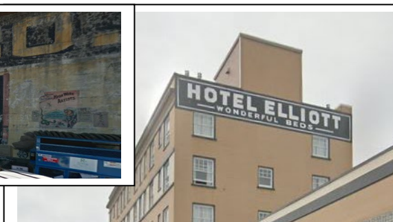
Hotel Elliott, 357 12 th Street - sign restoration
