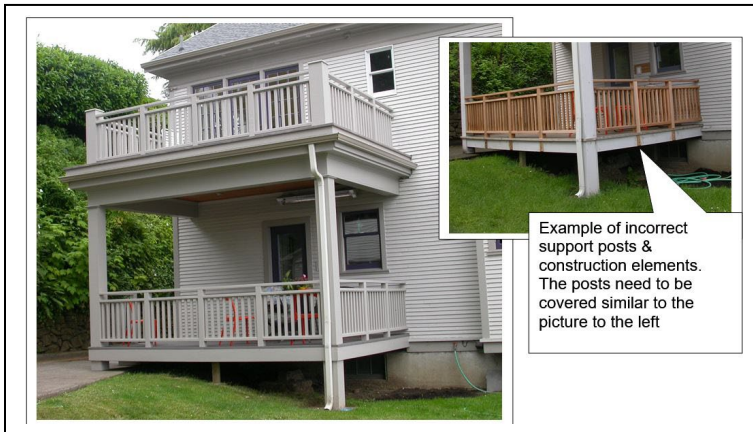
Example of balustrade construction
